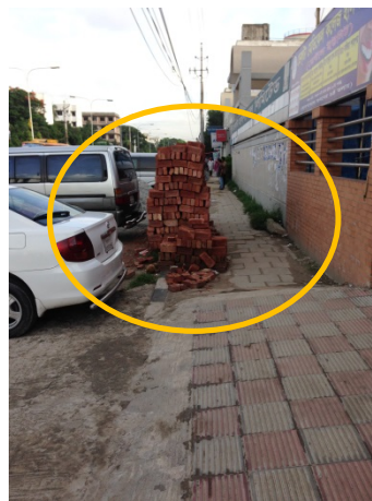
Construction materials on footpath
